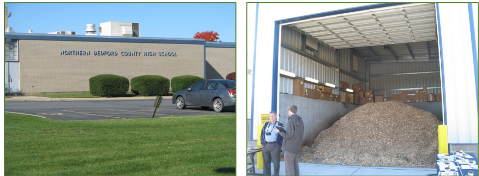
Northern Bedford High School (left) and their wood fuel storage bin (right).
