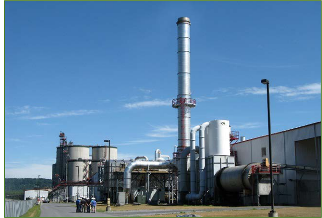
Starch (corn) based ethanol plants, like this one in Clearfield County, could serve as the starting point for advanced cellulosic ethanol production.
