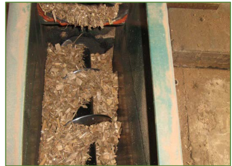
Dillon Floral's biomass boiler (top), greenhouse flowers (middle), and fuel being augered into boiler (bottom).
