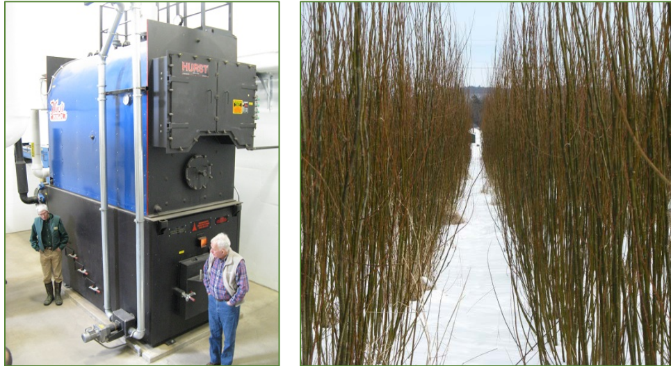
A view of the boiler at Hughesville high School (left) and looking down a row of shrub willow (right).
