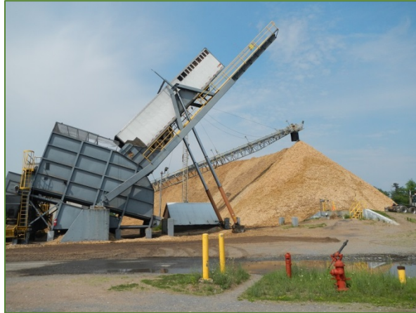
Wood-fired power plants are not common in Pennsylvania, but can be found in other Northeastern states (Photo: Justin Heavey).
